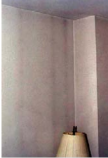
Particle deposition due to thermal bridging
