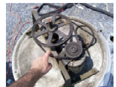
Ventilation fan belt adjustment
