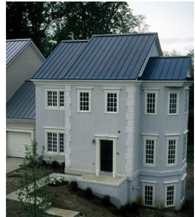
PV roofing system displaced traditional roofing materials
