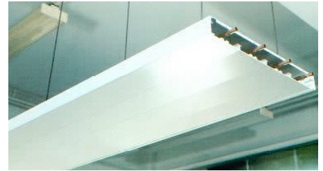
Examples of a ceiling panel radiator (above) and more intricate chilled beam (below)
