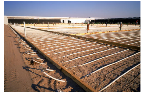
Radiant tubing for a greenhouse before slab is poured.
