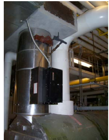
Motorized damper with draft controller
