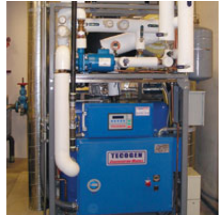
Commercial cogeneration unit
