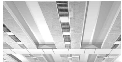
Examples of a ceiling panel radiator (above) and more intricate chilled beam (below)
