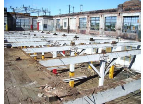
Deconstruction of a building
